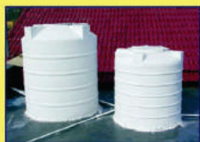
Heat Proofing on Water Tank
