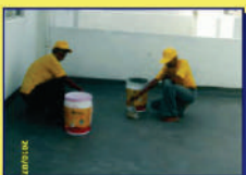
Multi Layer Coating on RCC
