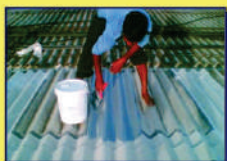
AC Sheet Repairing
