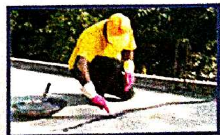
Fill Mixture In Crack
