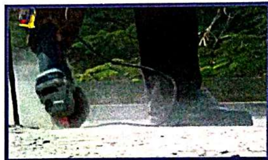
Grinder on Crack
