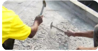
Removing Loose Material
