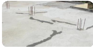
Fill Chemical in Cracks
