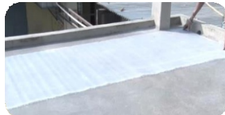
Laying Fibremesh
