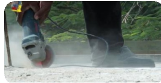
Opening Cracks in V Groove Shape
