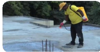
1st Coat Penetrative Waterproofing
